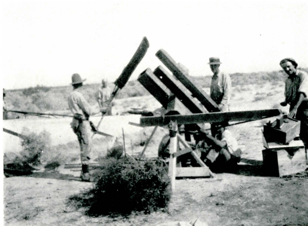
Figure 2. The "Combination" instrument with the crew at their places. This included a 15-foot equivalent focus, a 52-inch focus and a guiding telescope. The sector arm was driven by a Victrola motor.
